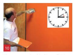
Mix a new quantity of A1 Plaster Finish and apply a 2<sup>nd</sup> layer onto the surface and level it. You can use the same or a different colour.
