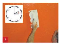
Use a stucco to create some structure (or any other tool) in the 1<sup>st</sup> A1 Plaster Finish layer. Processing time is max. 1 hour.
