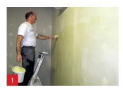
Make sure the surface is smooth. Then apply a stuc primer onto the surface.
