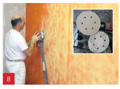
After curing (approx. 1 hour) lightly sand the surface with P80 sandpaper.
