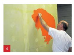
Apply a 1<sup>st</sup> layer of A1 Plaster Finish using a stucco and level it (approx. 1 mm thickness).
