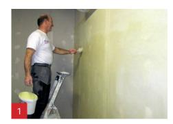
Make sure the surface is smooth. Then apply a stuc primer onto the surface.
