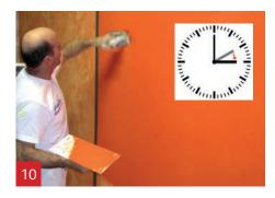
Mix a new quantity of A1 Plaster Finish and apply a 2<sup>nd</sup> layer onto the surface and level it. You can use the same or a different colour.
