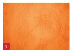
Result after sanding the 1<sup>st</sup> layer. Directly after sanding, the 2<sup>nd</sup> layer of A1 Plaster Finish can be applied.
