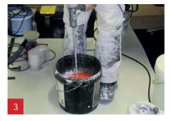
Mix Component B with Component A with the High Shear mixer till all lumps have disappeared (approx. 2 minutes).
